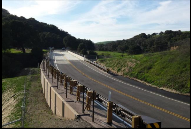
Jalama Road over Jalama Creek
